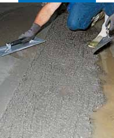
Screeding with mortar admixed with Idrosilex Liquid
