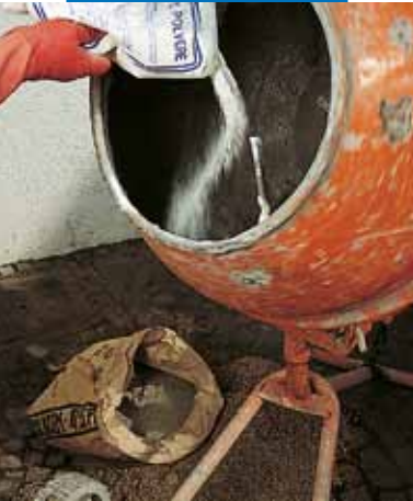
Preparing waterproof mortar admixed with Idrosilex Powder
