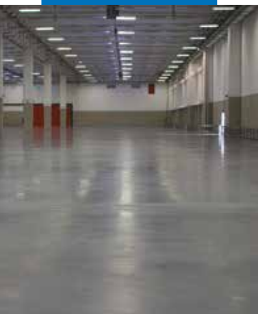
Example of industrial flooring admixed with Mapefibre NS12
