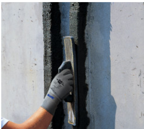
Finishing with a sponge float
