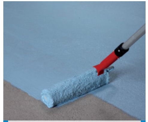
Application of the first coat of Mapelastac AquaDefense on a screed
