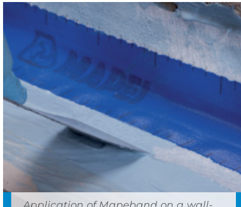
Application of Mapeband on a wall-floor fillet joint with Mapelastac AquaDefense
