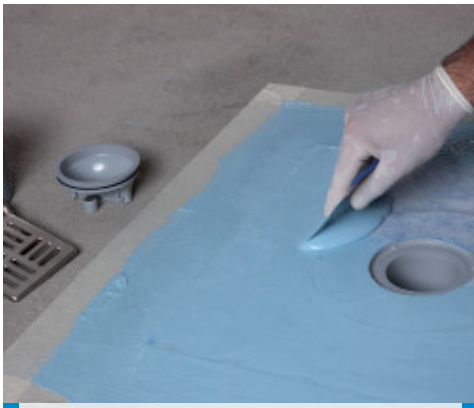
Impregnating Drain Vertical fabric with Mapelastac AquaDefense
