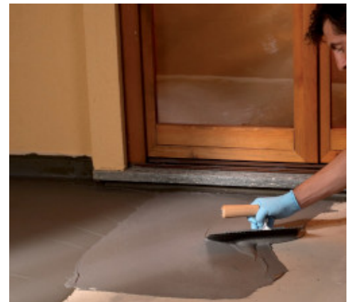
Waterproofing of terraces by trowel
