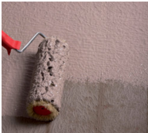
Waterproofing of details by roller
