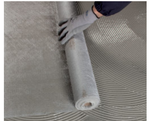
Placing Mapetex Sel N on the first coat of Mapelastic Turbo while till wet
