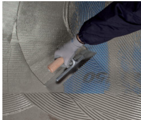
Placing Mapenet 150 on the first coat of Mapelastic Turbo while till wet
