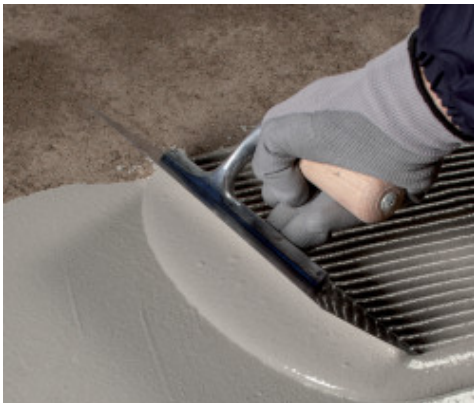
Application of the first coat of Mapelastic Turbo
