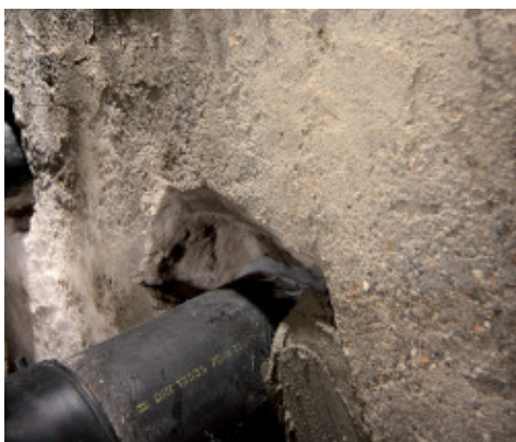
Confining Mapeproof Swell with a product of the Mapegrout line
