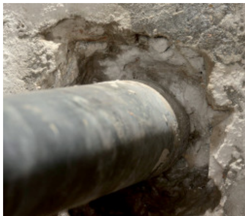
Breaking out structure around a pipe
