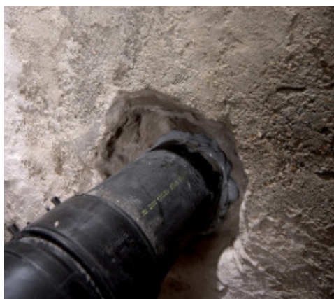
Mapeproof Swell after application
