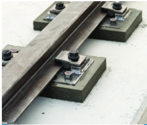
A detail of filling the gap under a support bed
