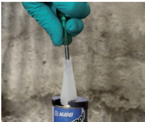
Piercing the protective membrane on the Mapeproof Swell tube
