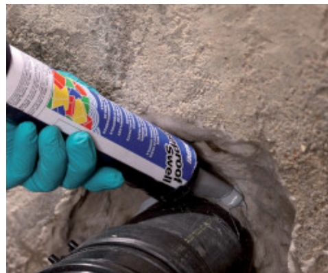
Applying Mapeproof Swell around a pipe
