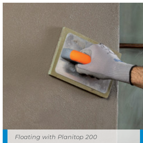
Application of the second layer of Planitop 200 on a substrate made from different materials with Mapenet 150 embedded between the layers
