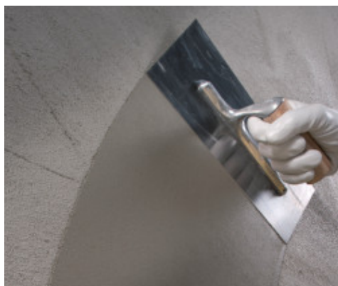
Applying Planitop 200 on concrete
