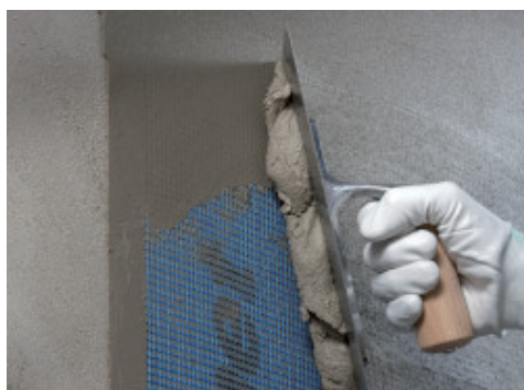
Application of the second layer of Planitop 200 on a substrate made from different materials with Mapenet 150 embedded between the layers
