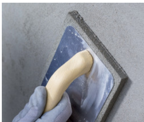
Floating the surface of Planitop Smooth & Repair R4
