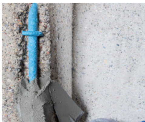
Applying Planitop Smooth & Repair R4 with a trowel
