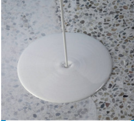
Application of Ultratop Stucco
