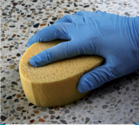
Dampening the surface with a sponge
