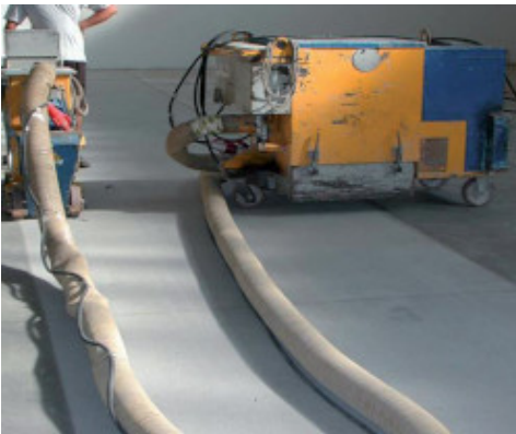
Preparation of the substrate by shot-blasting
