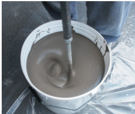
Preparation of the product with a drill
