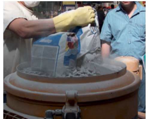
Preparation of Ultratop in a mixer
