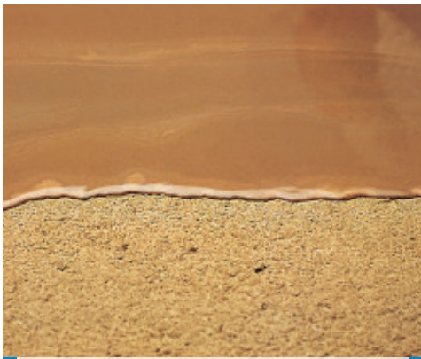
Finishing a Mapecem screed with Ultraplan self-levelling compound
