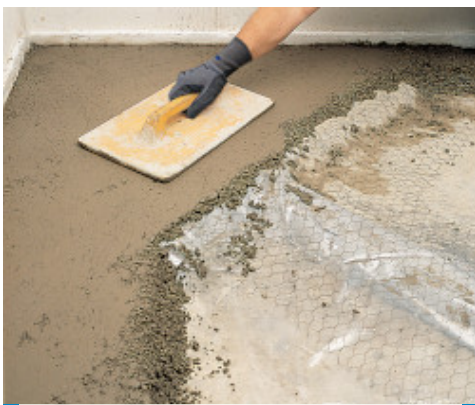
Covering pipes with Mapecem and reinforcement netting
