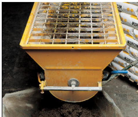
Mixing Mapecem in a mini-batcher
