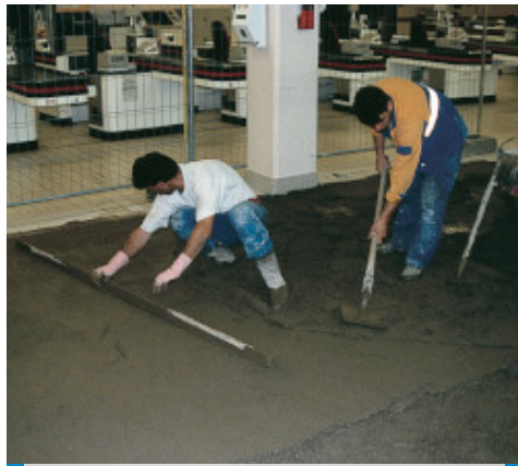
Tamping the Mapecem screed
