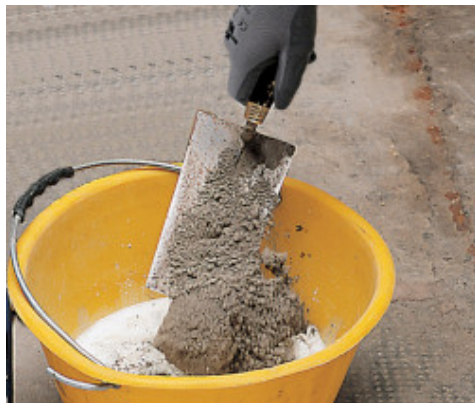
Mixing Mapecem with Planicrete to make an anchoring slurry
