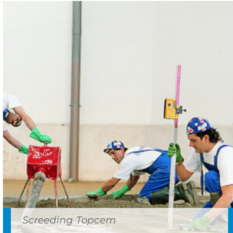
Mixing Topcem with an automatic pumping unit
